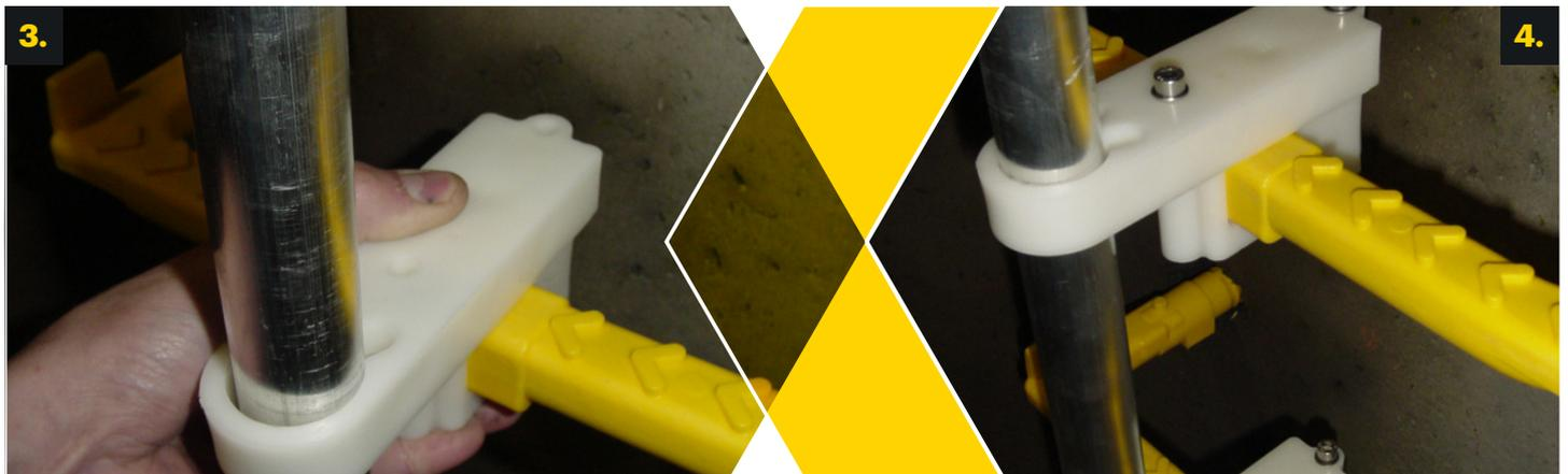
Fit upper half of bracket ensuring correct fit with step and lower half of bracket.
