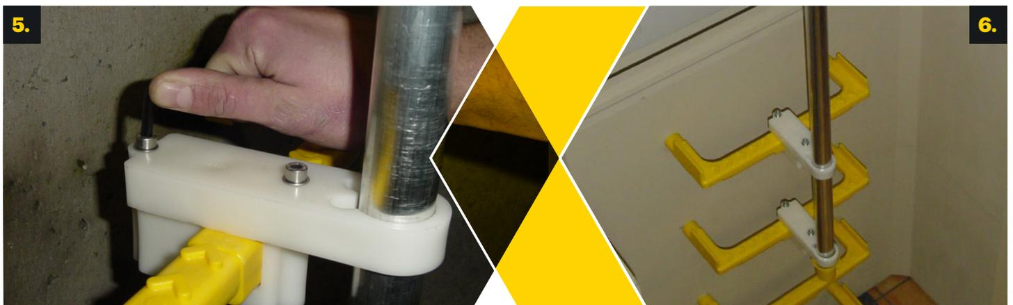
Tighten 4 screws with 5mm Allen key.
